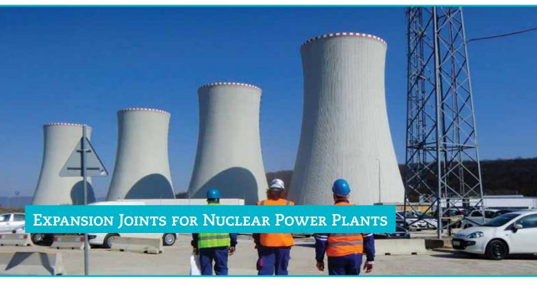
A large number of Lateral, Pressure **Axial** and Hinged Balanced, Expansion Joints from DN150 up to DN600 have been successfully manufactured and delivered to a European nuclear power plant.
